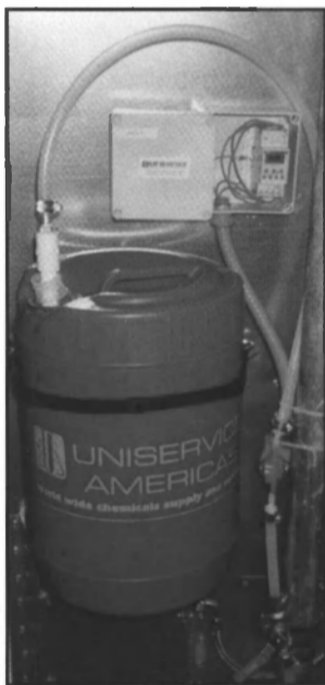
Uniservice's URICLEAN system was developed to help cruise ship owners avoid costly downtime due to problem build-up in a ship's sanitation piping system.
